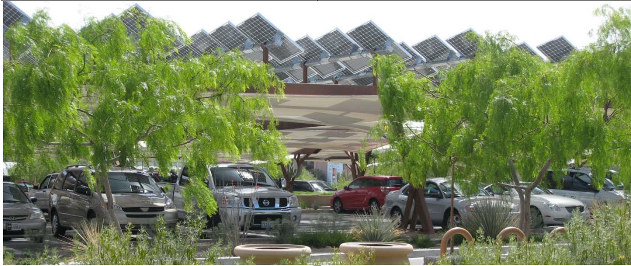
Photovoltaics over parking lot, Las Vegas.
